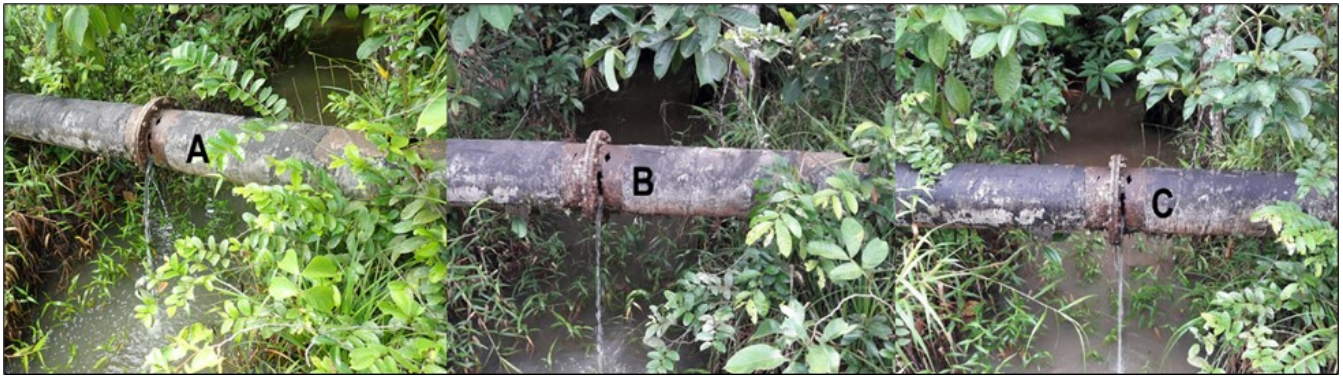
Figure 6. Observations of water spouting from an old WASA pipeline along the Old Railway Line, ASES, Trinidad. (A) August 2019, (B) October 2019 and (C) November 2019. Can you see the different floral families? (Arecaceae, Cyperaceae, Poaceae, Melastomataceae, Euphorbiaceae, Heliconiaceae, Apocynaceae, Orchidaceae, and Mimosoideae)
